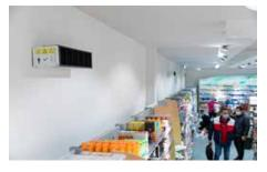
convection of airflow in the room. In this way, the maximum volume of air is disinfected, while at the same time safety is ensured and shoppers can continue to move about the stores. Pharmacy chain deploys upper-room UV-C lighting - Lux Review
